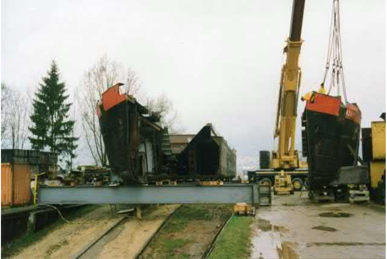
Construction yard in Arch. The fore ship is being assembled
