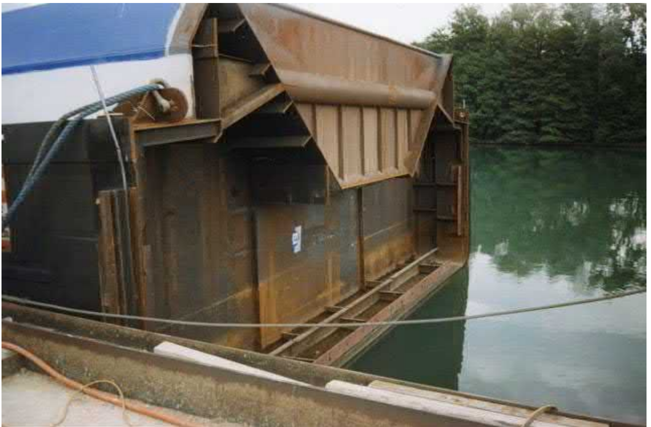
One of the sections, note the conveyor belt tunnel is temporarily closed-up with a steel plate
