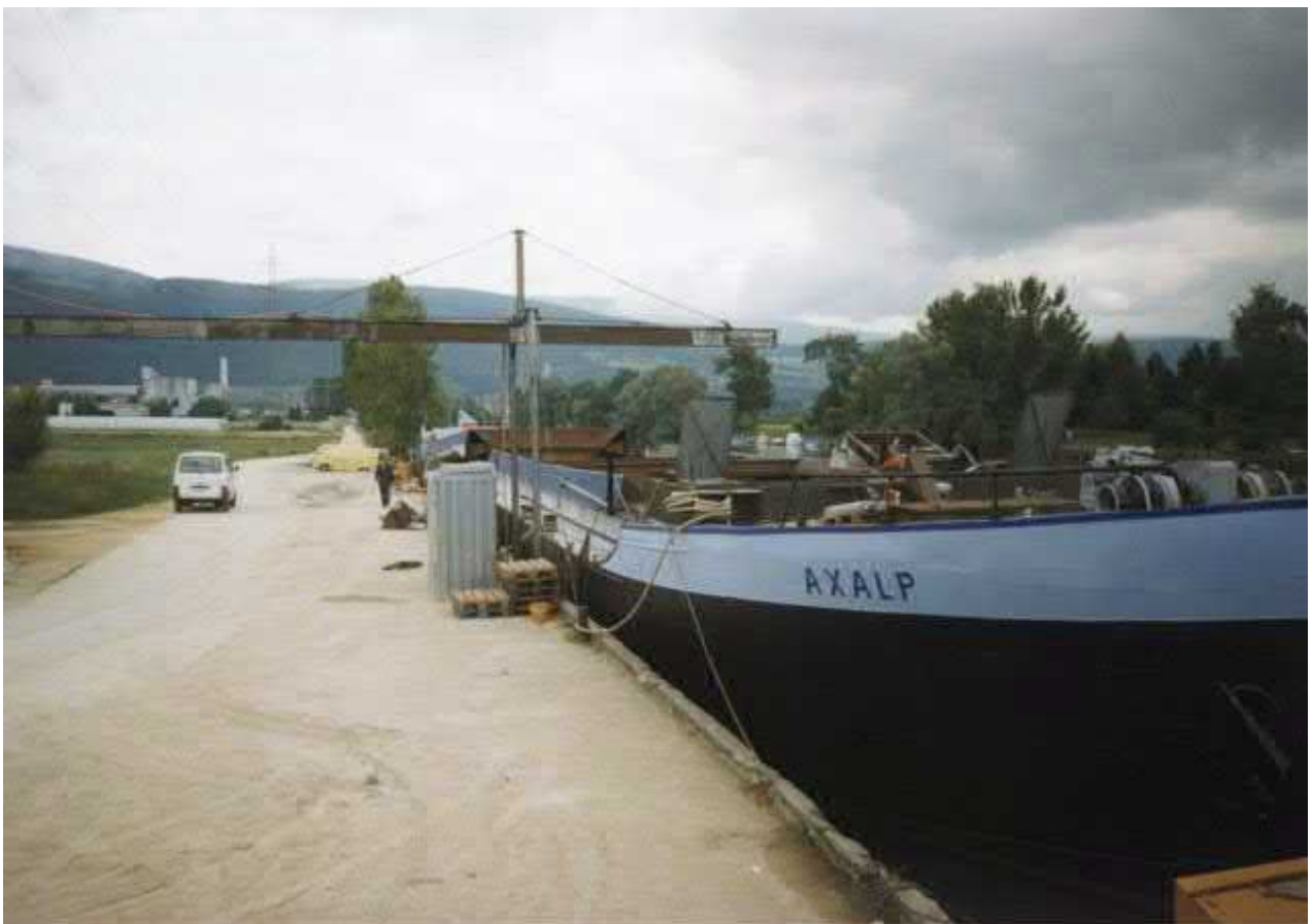
In the Zihl Canal at Thielle, ready to join the fore ship and the stern part Photo: © Uwe Mayer / Marti AG
